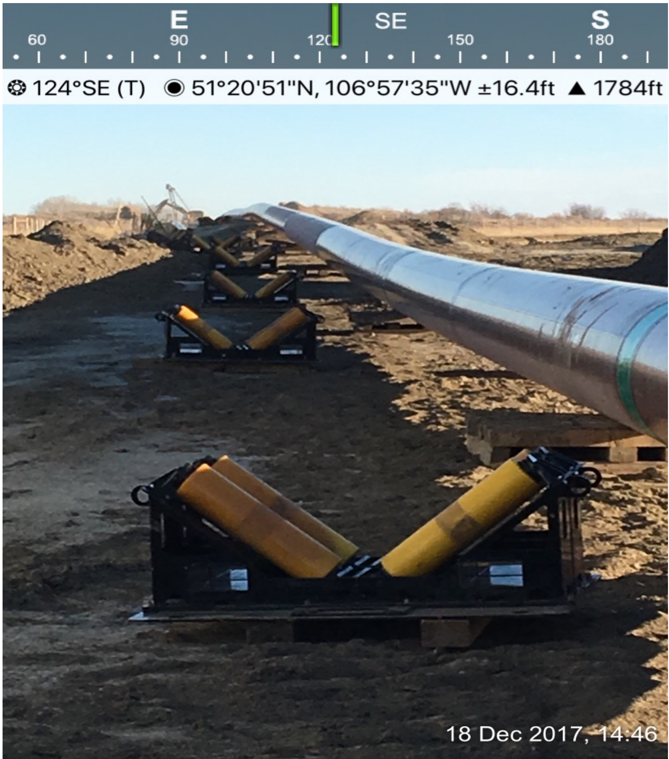
INSTALLING ROLLERS ON THE BORE SECTION
