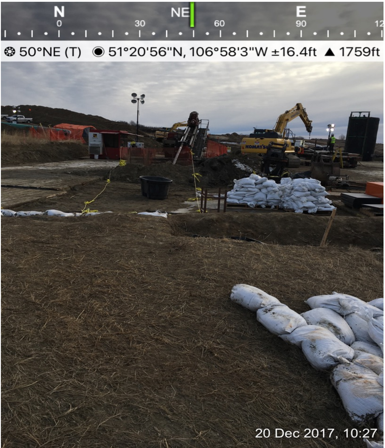
EXIT POINT OF HORIZONTAL DIRECTIONAL DRILLING
